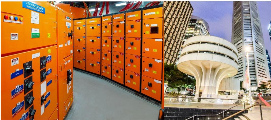
*The new Fuji SMBE Macquarie Switchboards (left) were modular in construction to fit into the curvature and tight confines of the room at the MLC Centre (right)*
